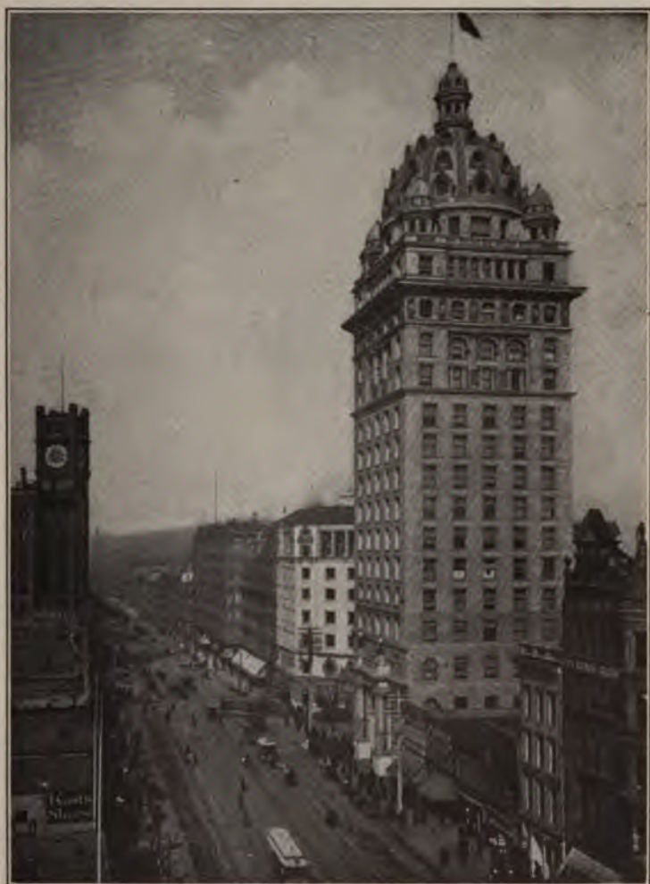
VIEW ON MARKET STREET, SAN FRANCISCO, SHOWING CHRONICLE BUILDING AND SPRECKELS BUILDING
